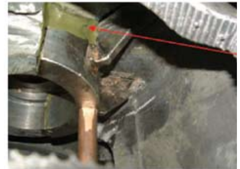
Insert in position with steel brackets.
