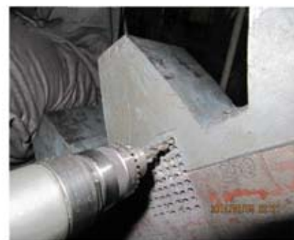
Master Keys were used to strengthen the repair.
