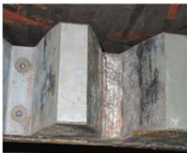
The two joints were welded together.
